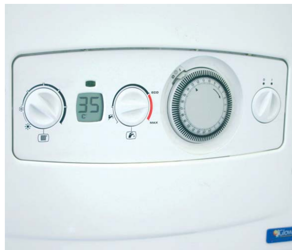
Control panel on boiler
